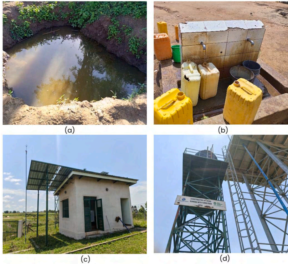
Fig. 2. Sources of water access: (a) Water stream; (b) Tap stand point; (c) Main diesel-solar hybrid station of the motorized solar tap water supply system; (d) 10,000 to 112,000 litres water reservoir tank for the motorized water supply system.
