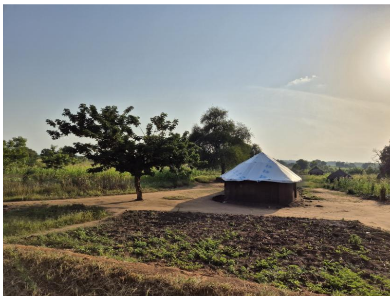
Figure 40: Plot of land divided into an area for the shelter and a garden.
